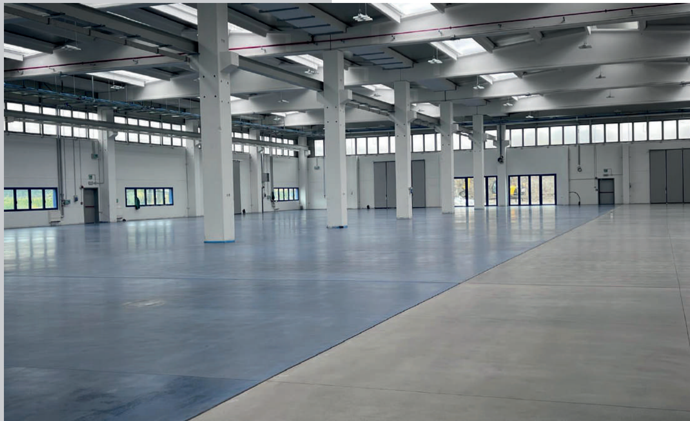
Colour-polishing of a warehouse.
