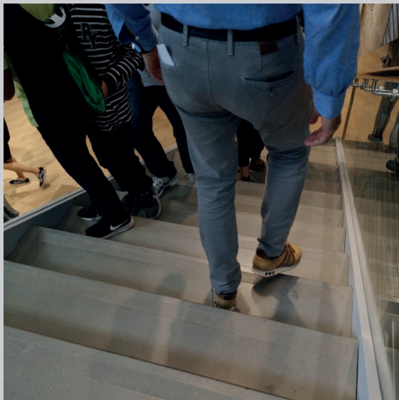
Pre-cast steps with Prima Polishing Concrete Floor finish Nike Stores Europe
