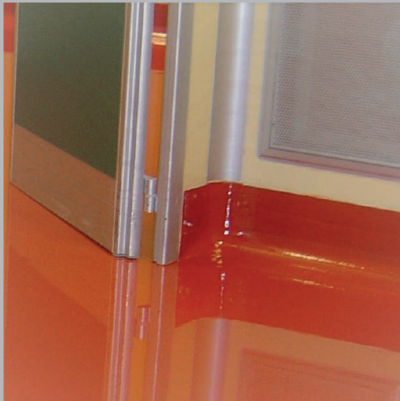
Floor-to-wall connection
