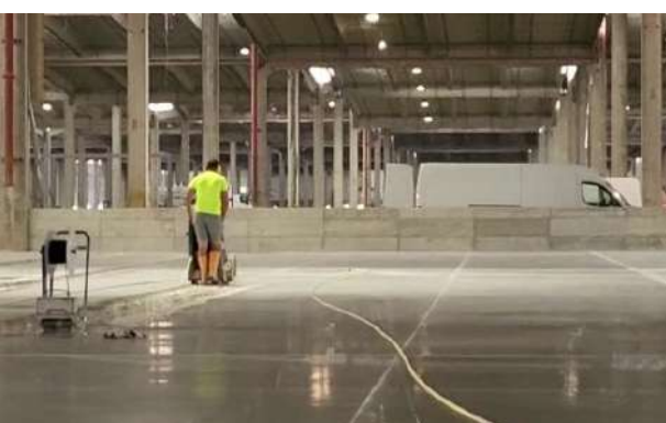
Control joint construction by cutting
