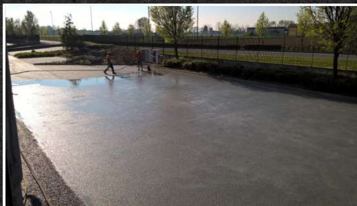
Asphalt clogging with cement mortar
