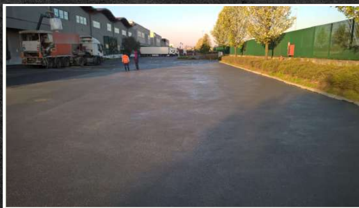
View of new applied asphalt
