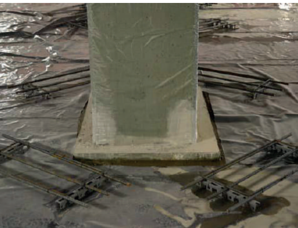
Laying of a vapour barrier consisting of 200-micron-thick polyethylene sheets.
