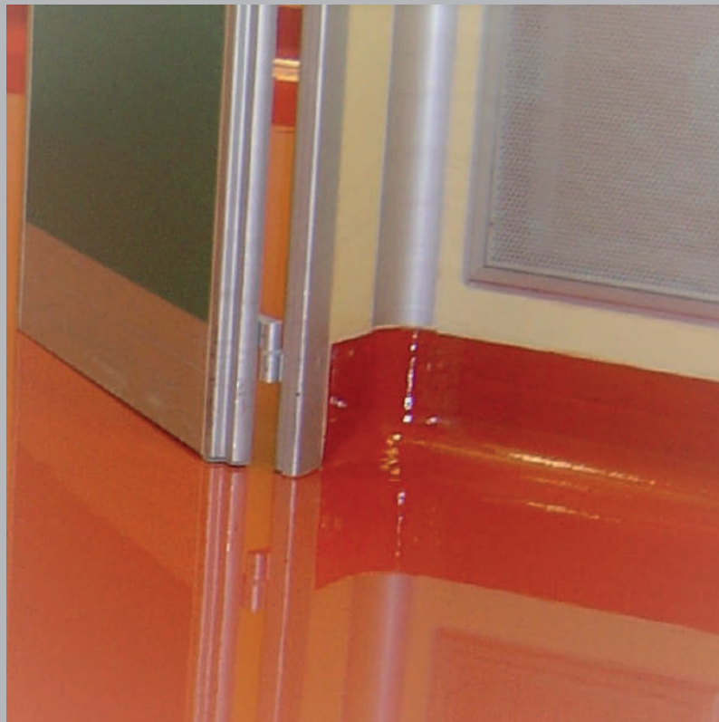
Floor-to-wall connection
